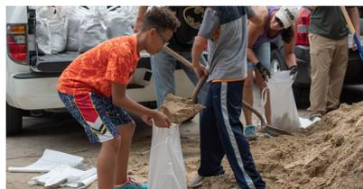
Sandbags can redirect stormwater and debris flows away from homes and other structures if they are correctly filled, placed and maintained. However, sandbags will not seal out water, and residents should not rely on sandbags to save their home from major flooding, especially fast-moving hurricane storm surge flooding. Consider the severity of
